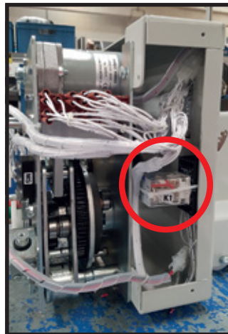
5- Anti-Pumping Relay
